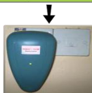
ELCB box / Distribution Channel
